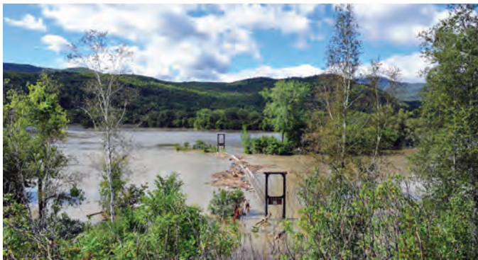
Debris catches on snowmobile bridge near Waterbury, Vermont, as a result of floodwaters from the Winooski River during Tropical Storm Irene, in August 2011. Photograph courtesy of Lars Gange, Mansfield Heliflight.
